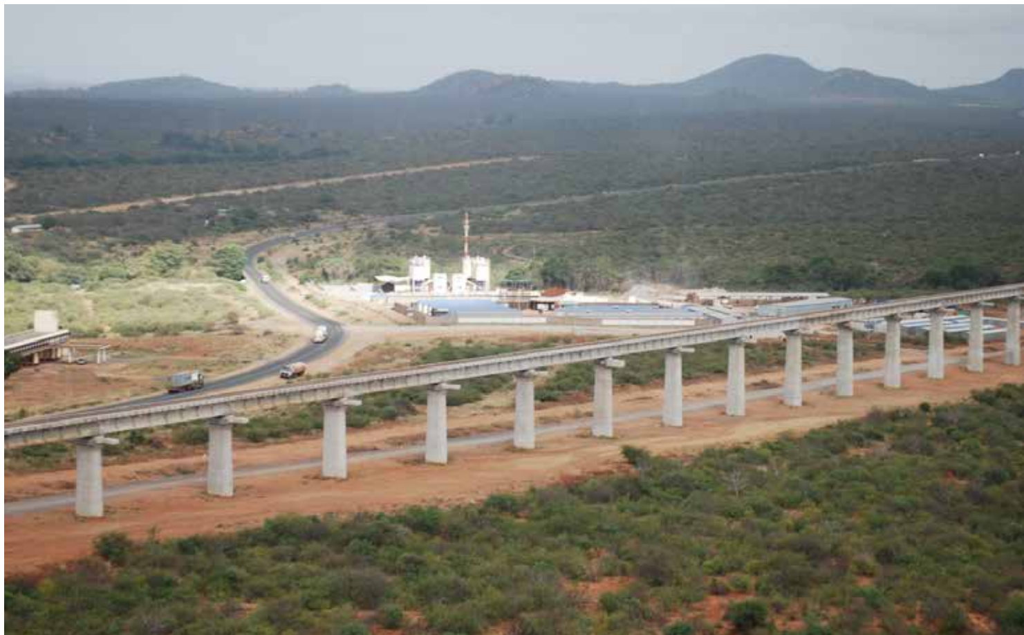
Plate 7.11: Aerial view of the SGR Tsavo River super-bridge, with underpass for use by wildlife. Next to it is the Mombasa-Nairobi highway. An overpass allowing animals to cross the highway needs to be urgently considered. Photo: courtesy Richard Moller/Tsavo Trust.
