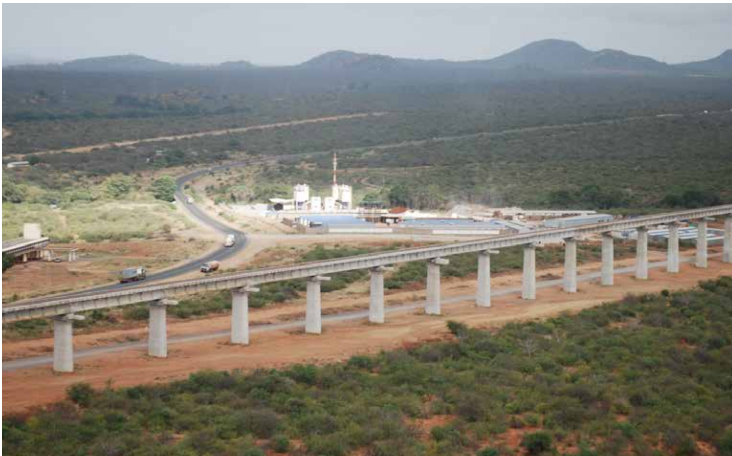
Plate 7.11: Aerial view of the SGR Tsavo River super-bridge, with underpass for use by wildlife. Next to it is the Mombasa-Nairobi highway. An overpass allowing animals to cross the highway needs to be urgently considered. Photo: courtesy Richard Moller/Tsavo Trust.
