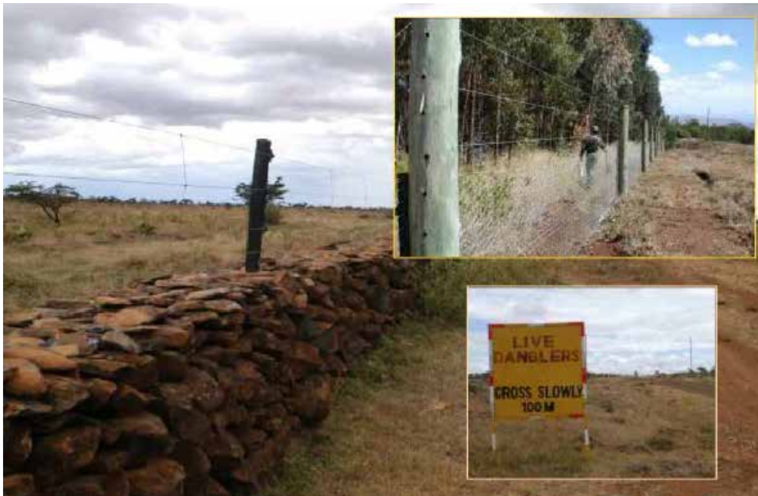
Plate 7.9.8(b): Types of the fences on some ranches and conservancies in the Laikipia landscape include combo stonewall/electric fences, chainlink cum electric fences (top inset), and live danglers across motorable pathways (bottom inset). Photo Courtesy: Gordon Ojwang.
